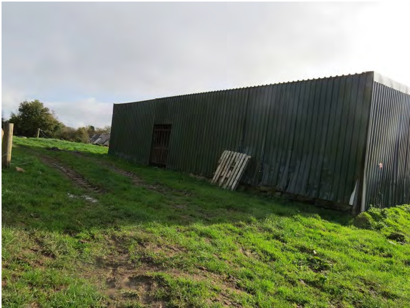
Figure 2.1 Existing Agricultural Structure to North of Site
